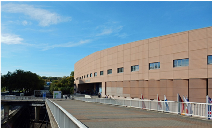
A view of the West entrance with the train tracks down below
