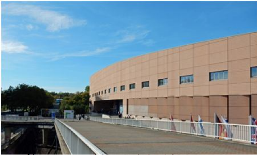
A view of the West entrance with the train tracks down below
